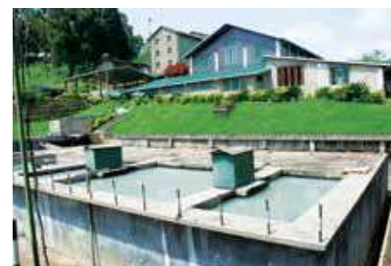
Effluent treatment plant - Panawatte
